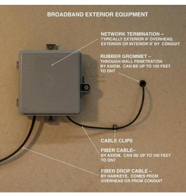
Axiom's Outside Plant Contractor will bring the fiber cable from the street to your house. Once the fiber is at your building, they need to mount a small plastic box (a Network Interface Device "NID") to terminate and test the new fiber.
