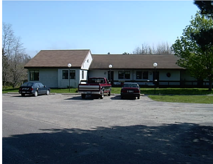
Atlantic Apartments on Swan's Island
